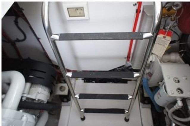
Engine room entrance
