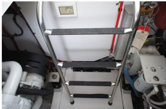
Engine room entrance
