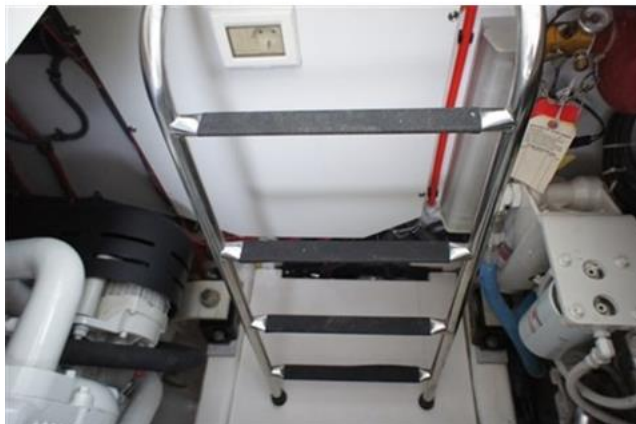
Engine room entrance
