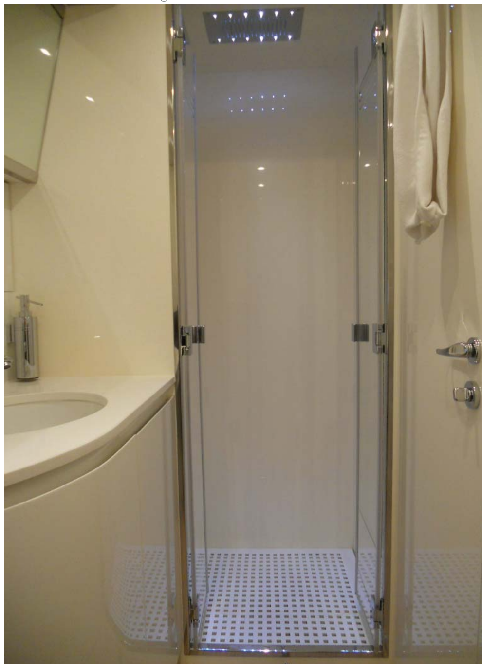
Doccia bagno armatoriale - Owner bathroom's shower
