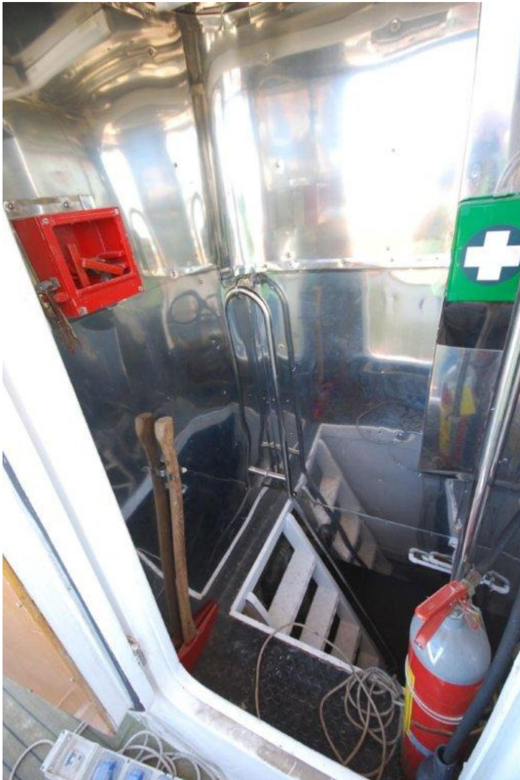
Engine room entrance
