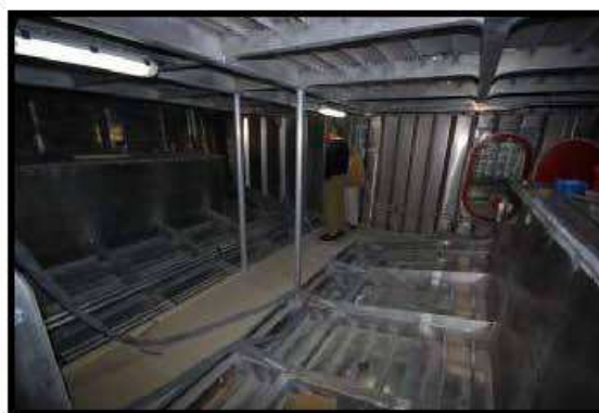
Fuel tank view
