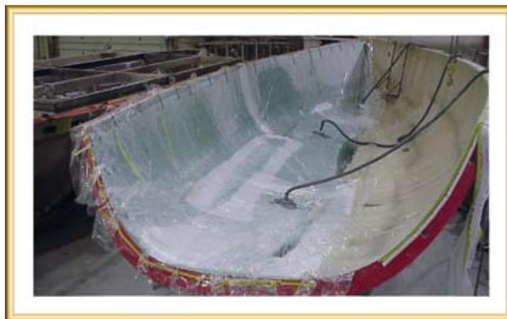
Vacuum-bagging the hull
